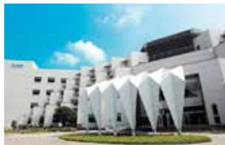
Tainan Plant (Diamond-rated Green Building)
