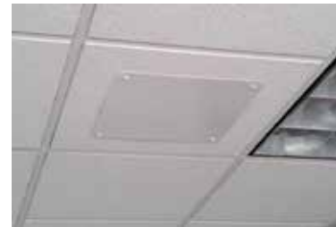
Installed Condition: PSIBVHF and PSIBVU78
