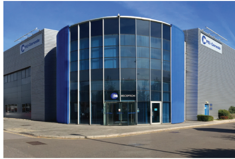
European Headquarters & Production Facility, Southampton, UK
