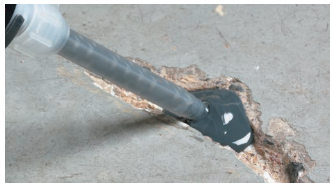
50mL and 400mL duo-pak cartridges are available to meet your production volume requirements. Nozzle automatically and precisely meters, mixes, and dispenses two-part urethane formulation. Apply material precisely where needed to conserve material.
